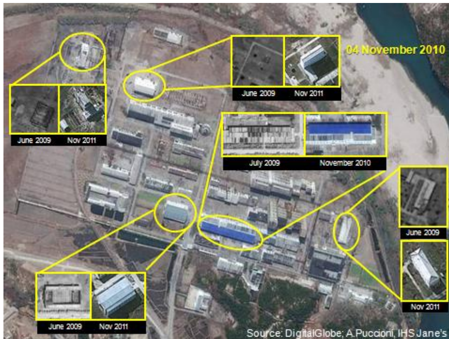
Figure 5 – The fuel fabrication plant in November 2010, with annotations identifying newly constructed buildings on the site between June 2009 and November 2011
