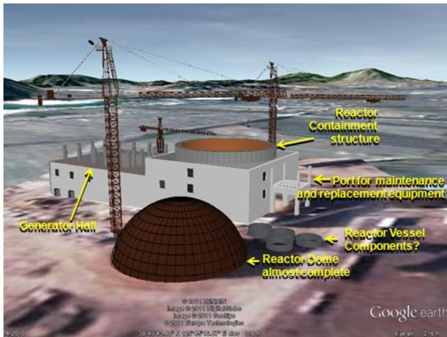
Figure 3 – Three-dimensional model of the light water reactor based on latest satellite images
